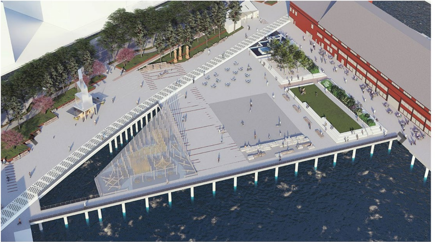
Pier 58 will be rebuilt in a triangular shape, with an opening in the nearshore to improve salmon habitat. The overall square footage will remain approximately the same as the current pier.
